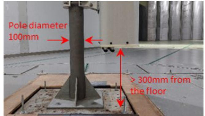
Figure 6: Installation requirement
