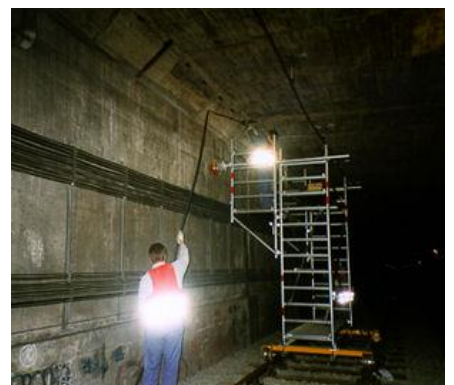
with movable scaffold,
