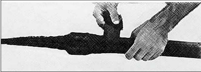
3. Wrap the connection with a layer of 2" black electrical tape and then the 3/4" black electrical tape. Overlap each tape a half-width and wrap 1" beyond the rubber tape. Do not pull and tear the tape during the last few turns. Tape should be cut in order to prevent unraveling.
