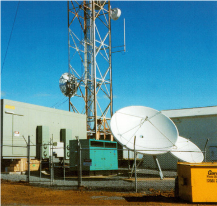
Fig. 2: Shared free to air and pay-TV installation at Shepparton (Victoria). The 19 channel headend uses 50W Comwave transmitters and supplies signals via 1-5/8" feeders to a dual input antenna mounted at the 60 metre level. Program is received via satellite (KU and C Band) and emergency power from a 60KVA standby generator.
