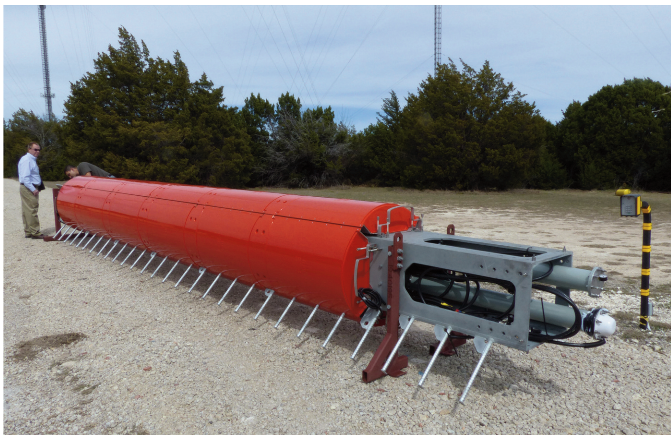
March 2016 Pre-installation inspection of PEP-Lite low wind load, broadband pylon alternative antenna on site at Cedar Hill Texas. (Photo courtesy of Jim Stenberg with American Tower)
