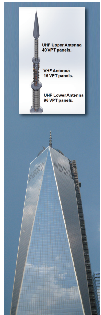
Freedom Tower At One World Trade Center, RFS is installing three antenna arrays with Variable Polarization to support multiple broadcasters' coverage requirements for New York City.
