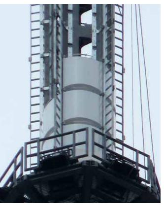
PEP40 UHF Antenna showing adapter plates and new External Climbing System – Photo Credit: © Tony Fonseca 2016
