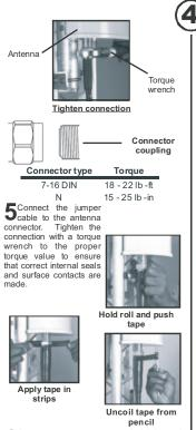
6 Start wrapping three layers of 3/4" (19mm) plastic tape 1" (25mm) at the connector clamping nut, overlapping at half width. The tape should extend 1" (25mm) beyond the cable connector clamping nut.
