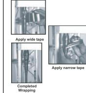
8 Wrap two layers of 2" (50mm) plastic tape and then three layers of 3/4" (19mm) plastic tape to complete the wrapping. Start each wrap 1" (25mm) from the previous wrap
