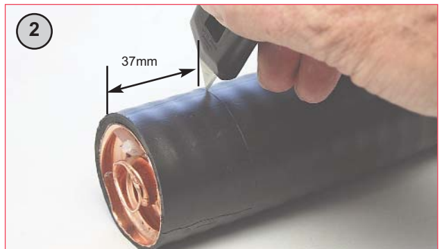
Trim jacket and outer 37mm (1 7/16") carefully, using a knife or hacksaw, ensure copper outer is not scored or cut.
