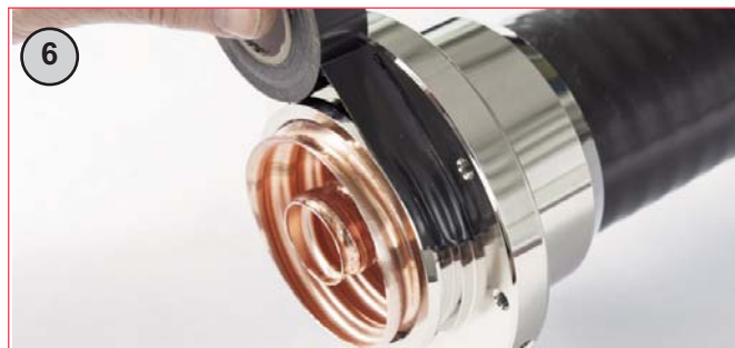
6 Remove O-ring and protect groove with PVC tape.
