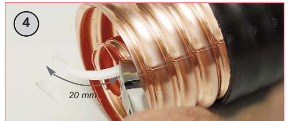
4 Trim and discard 20mm (3/4") off the helix then push back into original position. Make sure copper inner & outer edges are smooth and free of burrs and copper surfaces are clean, using the file and scouring pad. Ensure all debris is removed.
