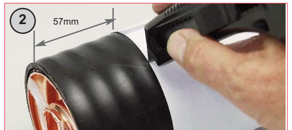
2 Trim jacket 57mm (2-1/4") carefully, using a knife or hacksaw, ensure copper outer is not scored or cut. NB: A piece of paper makes a handy guide.
