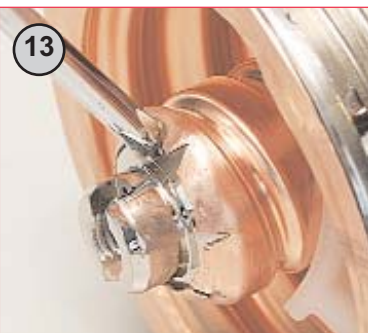
Indent cable inner conductor to prevent connector inner nut from rotating.
