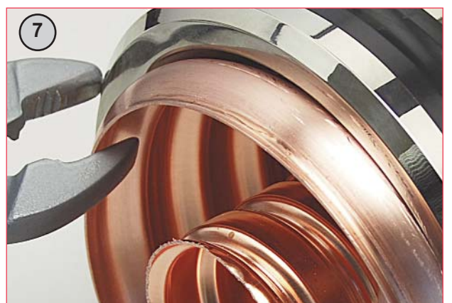
7 Flare outer conductor with soft jaw pliers. Work slowly around the perimeter flaring a small amount each time. Do not split the copper (refer Step 15 for remedial process).
