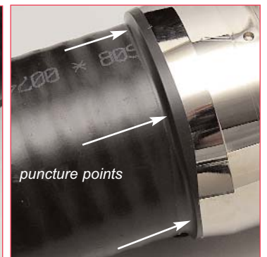
19 Remove both screw caps on back nut. Finely spray back nut/cable with water to accelerate curing. Inject sealing compound (approx 250cc) until the sealant appears at the opposite side of the back nut. Replace cap to stop further flow of sealant. Wrap insulating tape around the rear of the back nut/cable. Puncture the tape in 4 places as shown and then continue injecting compound until it appears at the puncture points. Remove sealant tube cartridge and replace screws. Do not pressurise for 24 hrs to allow compound to harden.
