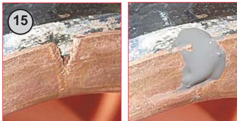
15 In the unlikely event that the outer conductor has split or torn, repair by adding Pactan sealant as shown allowing 45 min to set before fitting the connector body to the back nut.
