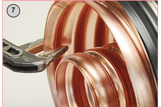
Flare outer conductor with soft jaw pliers. Work slowly around the perimeter flaring a small amount each time. Do not split the copper (refer Step 15 for remedial process).
