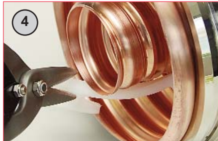
Pull out approximately 50mm (2.0") of helix. Trim and discard approximately 40mm (1 1/2") off the helix then push back into original position. Make sure copper inner & outer edges are smooth and free of burrs and copper surfaces are clean, using the file and scouring pad. Ensure all debris is removed.
