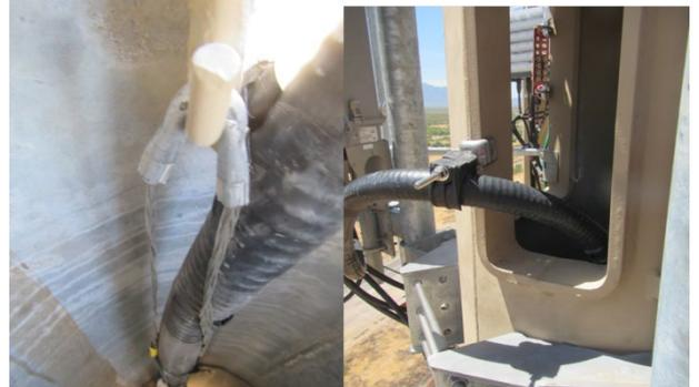
Once the hybrid cable is hoisted to the appropriate height, anchor it to the support structure, starting at the top.
