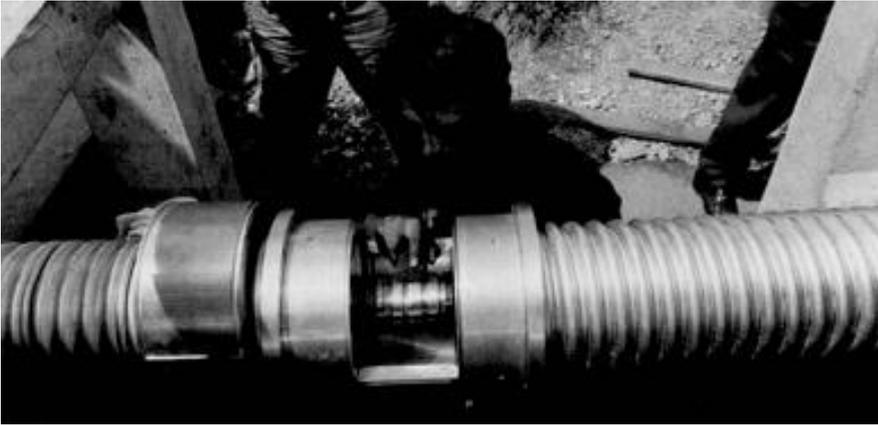
Fig. 4: View of a cable Coupling for Type HF9"-S AL Cable during Installation
