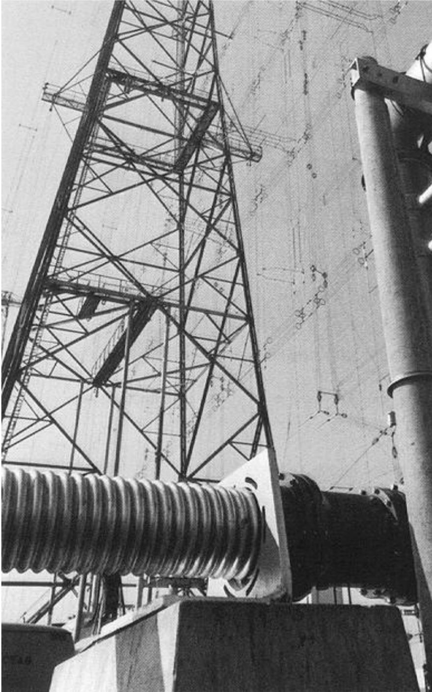
Fig. 6: HF9"-S AL type Cable connected to Coaxial/Symmetric Transformation Line
