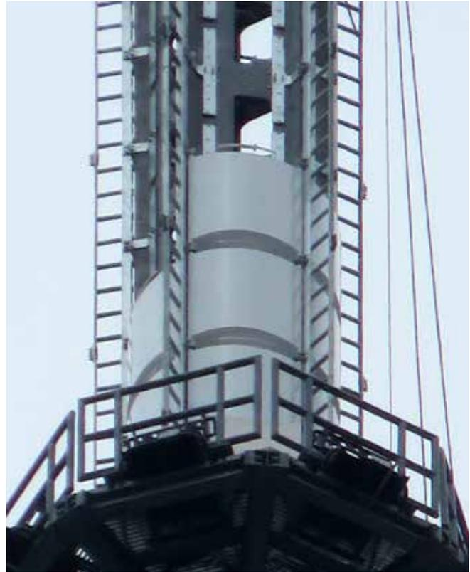
*PEP40 UHF Antenna showing adapter plates and new External Climbing System – Photo Credit: © Tony Fonseca 2016*
